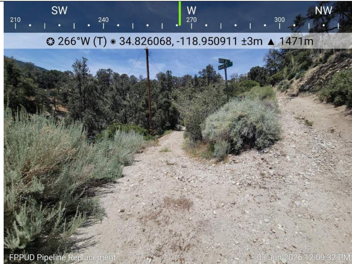
Photo 9. Replacement pipeline alignment within Manita Trail. North End Trail on the right, Oakdale Drive on the left.
