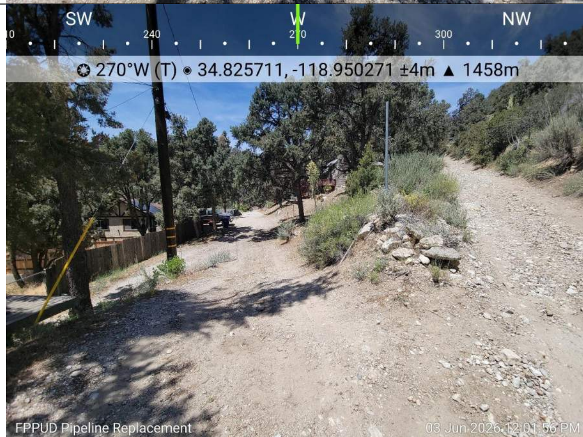
Photo 8. Replacement pipeline alignment within Oakdale Drive. North End Trail on the right, Oakdale Drive on the left.
