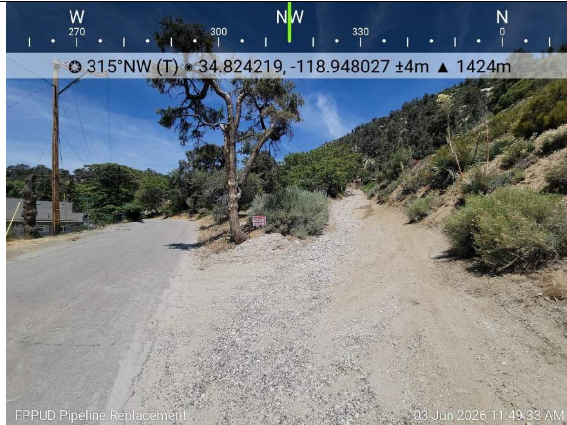
Photo 5. Replacement pipeline alignment within North End Trail. Los Padres Drive on the left, North End Trail on the right.
