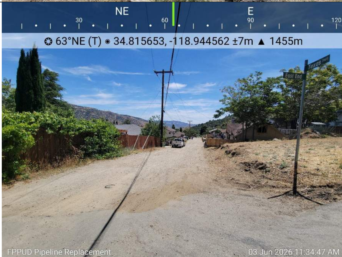
Photo 4. Replacement pipeline alignment within Texas Trail.
