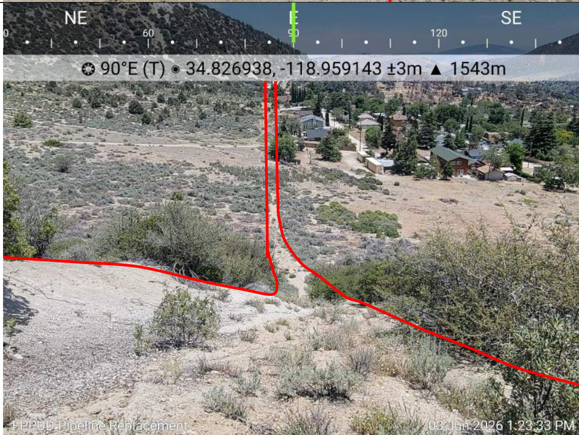
Photo 20. Replacement pipeline alignment between Elm Tank and McGhee Tank.
