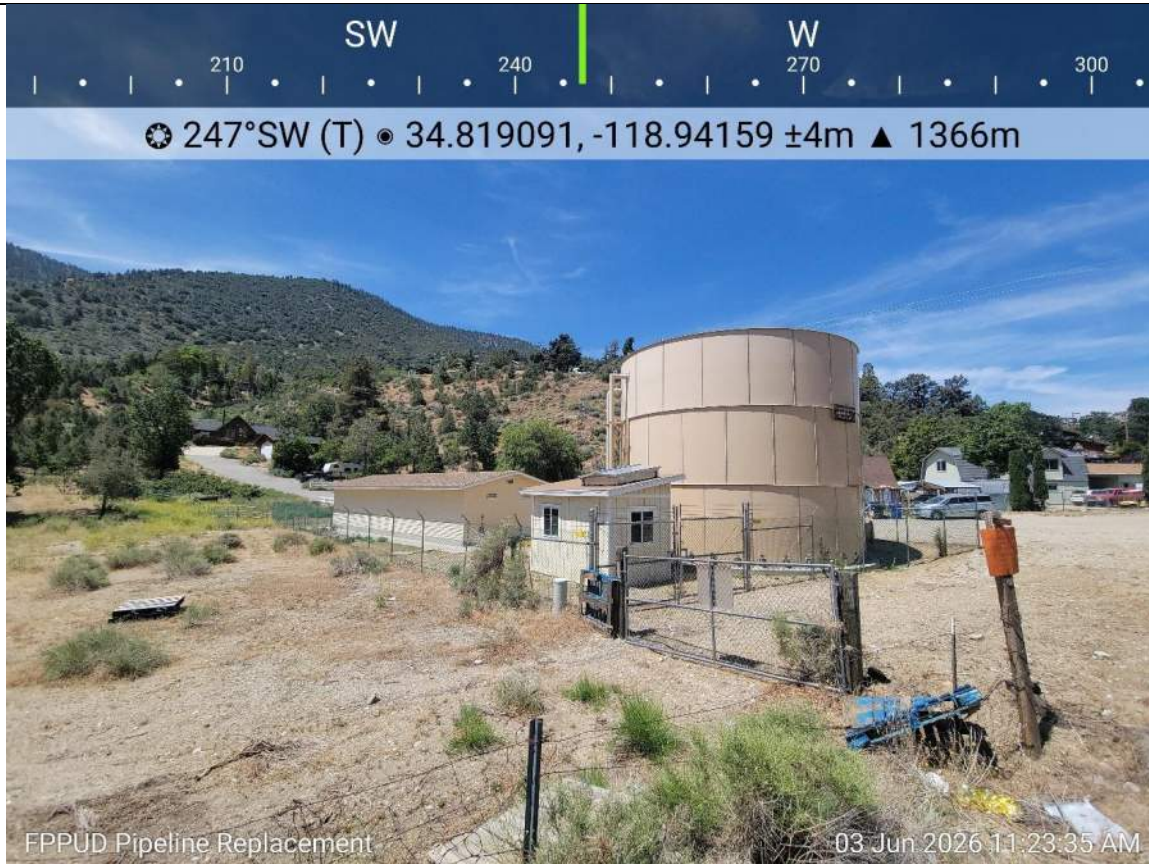
Photo 3. Existing Well #5 and storage tank site.
