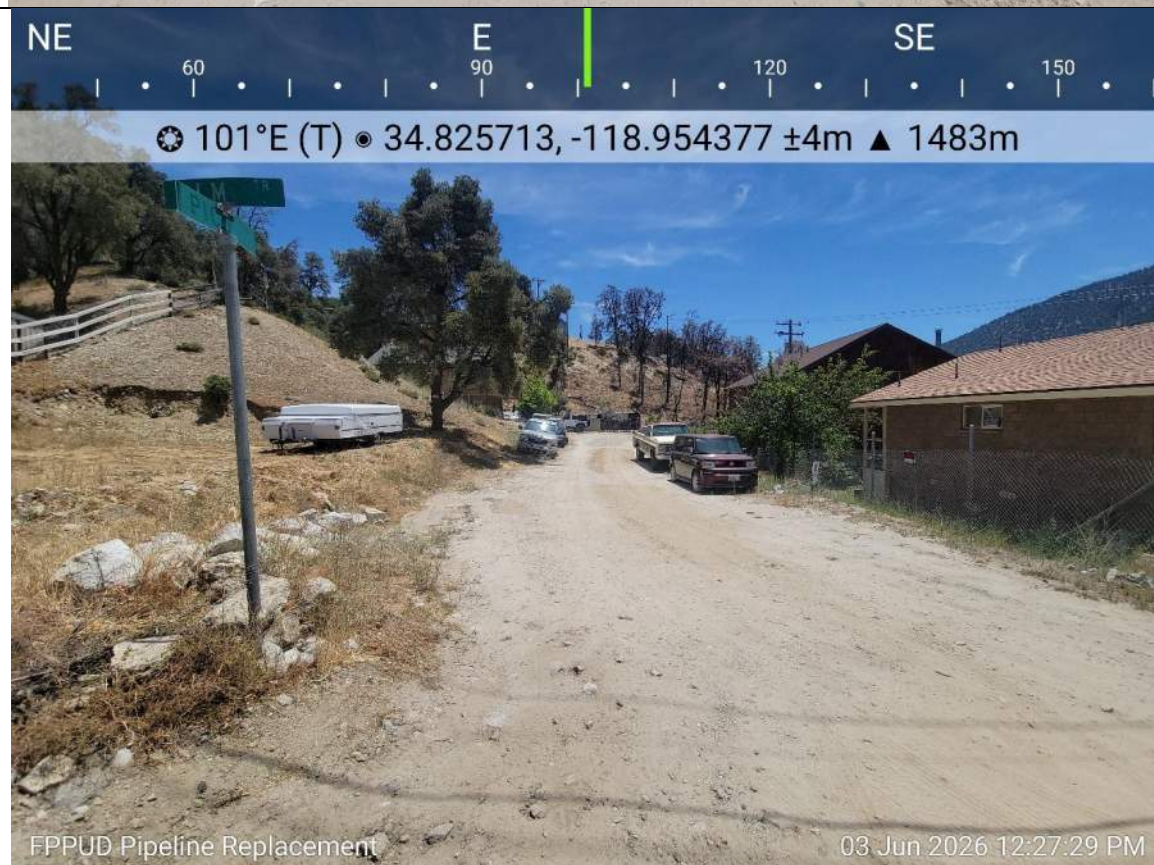
Photo 12. Replacement pipeline alignment within Pico Trail from Elm Trail.
