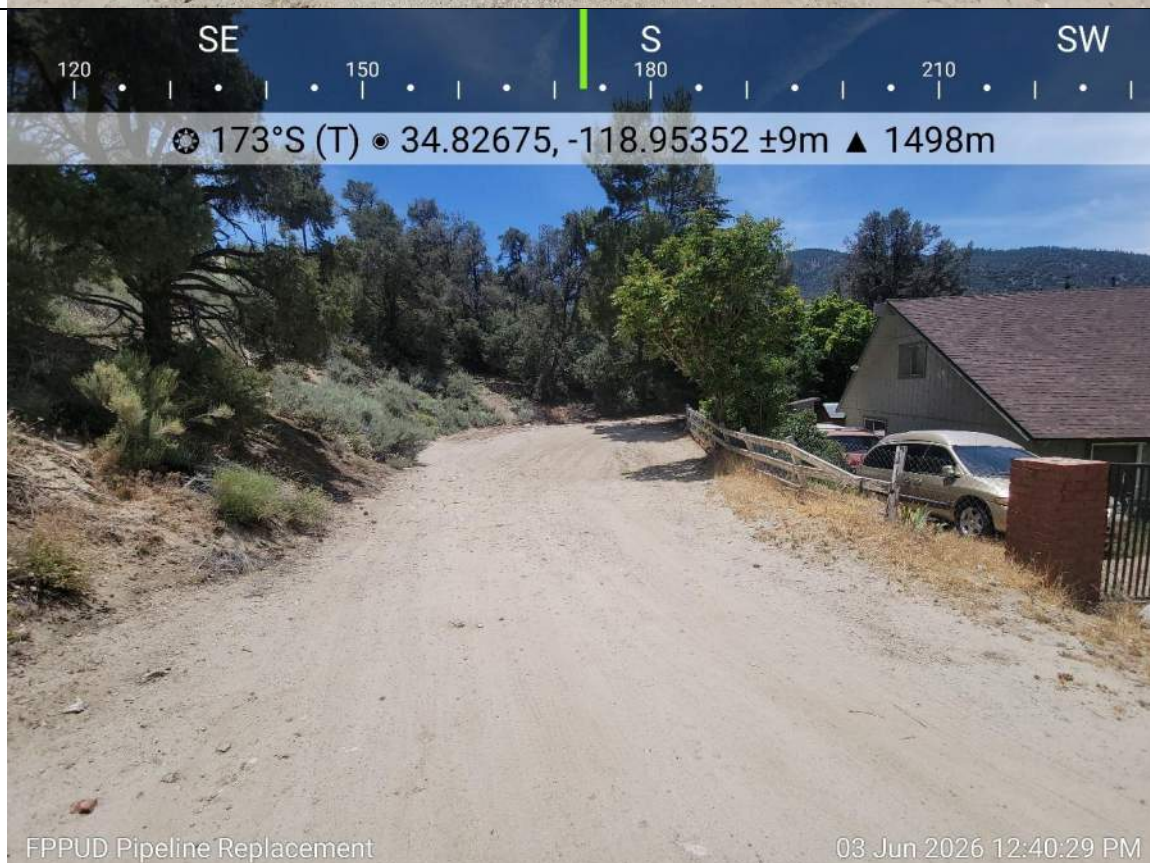
Photo 14. Replacement pipeline alignment within North Summit Drive from Elm Trail.
