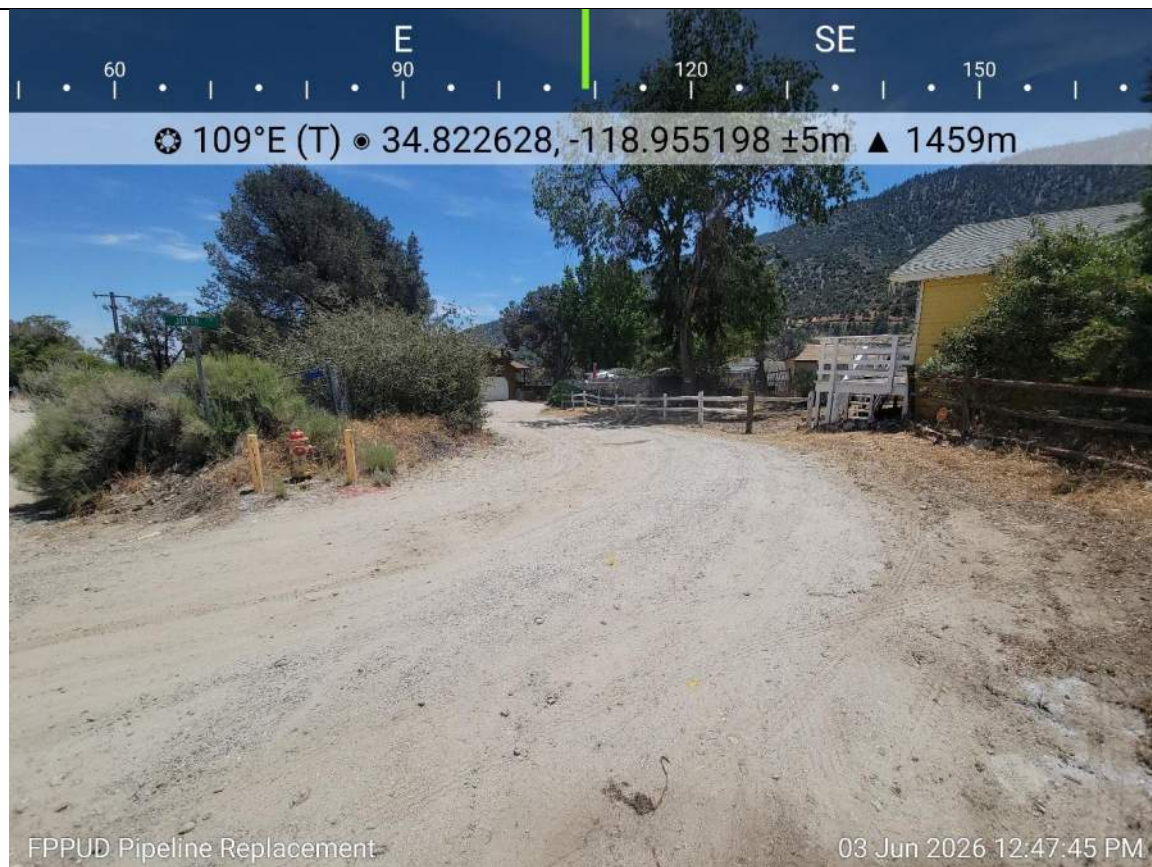
Photo 15. Replacement pipeline alignment within Julin Trail from Decator Trail.
