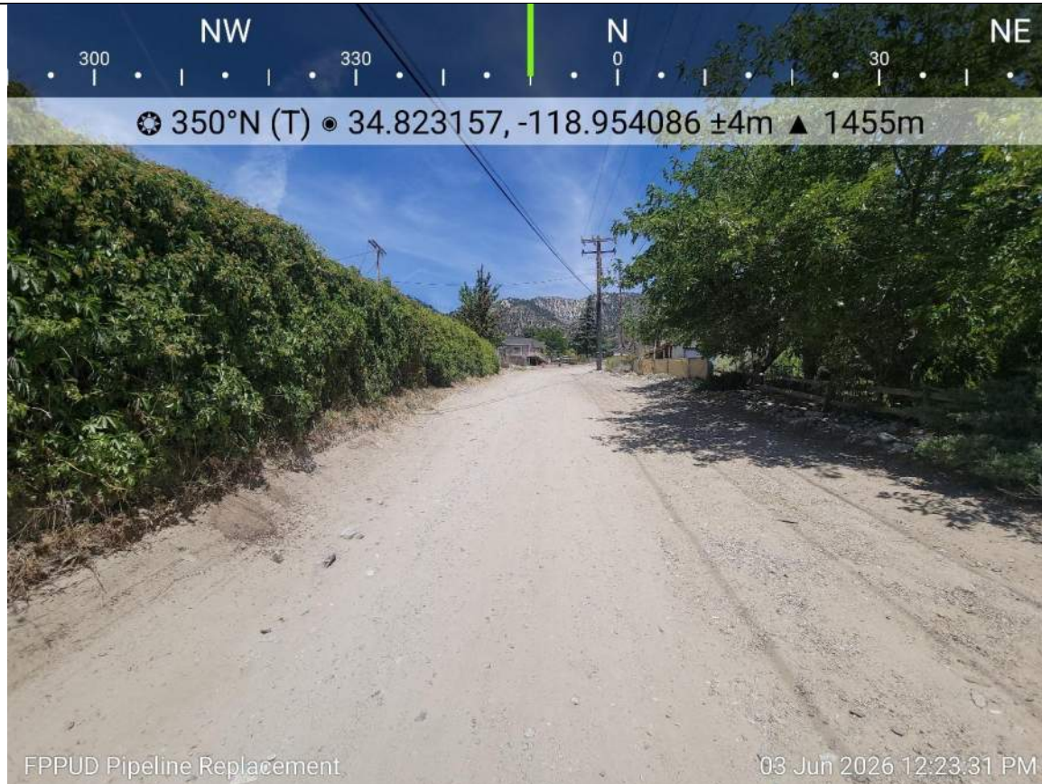
Photo 11. Replacement pipeline alignment within Elm Trail from Mt. Pinos Way.
