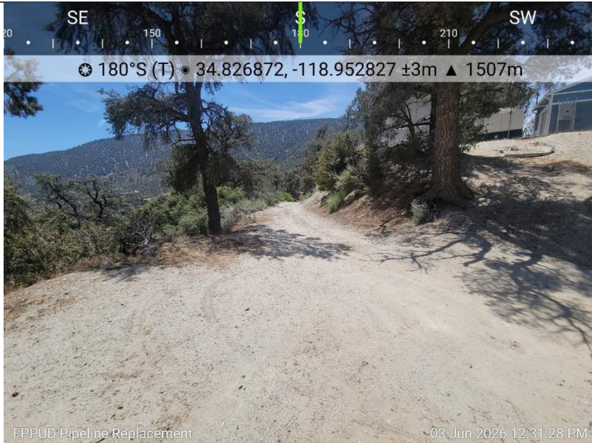
Photo 13. Replacement pipeline alignment within North Summit Drive from North End Drive. Existing Elm Storage Tank on the right.
