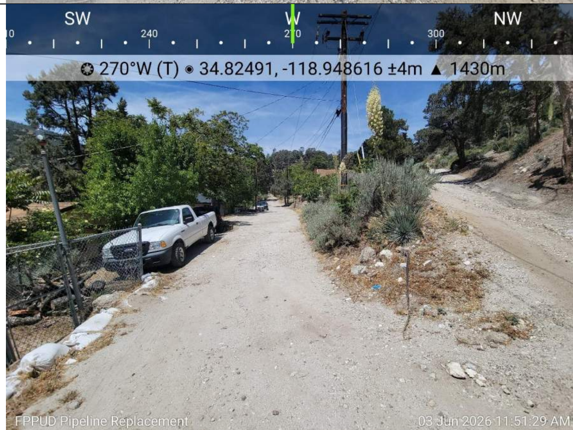
Photo 6. Replacement pipeline alignment within Laurel Avenue. North End Trail on the right, Laurel Avenue on the left.
