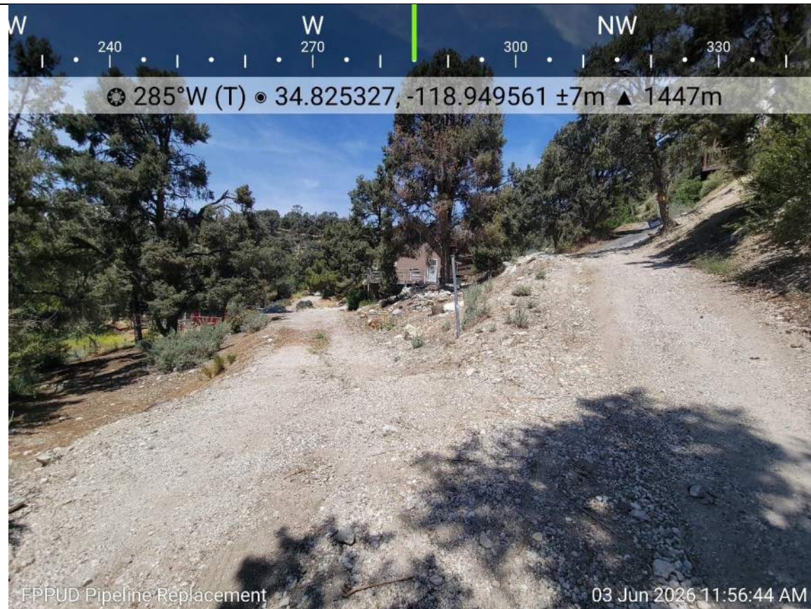
Photo 7. Replacement pipeline alignment within Oregon Drive. North End Trail on the right, Oregon Drive on the left.
