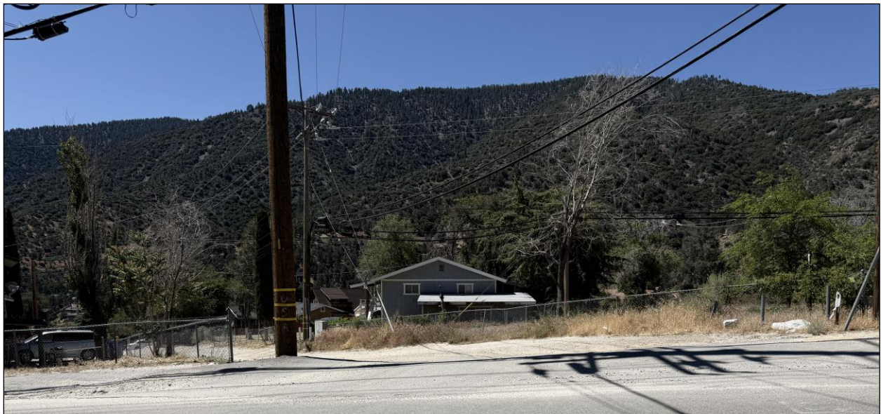
Figure 11. Wooden power pole of the Frazier Park-Gorman 66kV Transmission Line at Mt. Pinos Way and Elm Trail (Site 15-020579), view to the south. (Photograph taken on May 19, 2026)
